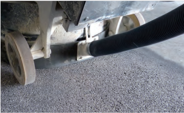
Machine scarifying the subsurface
