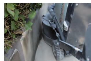
Grinding close to the edge with the remote control
