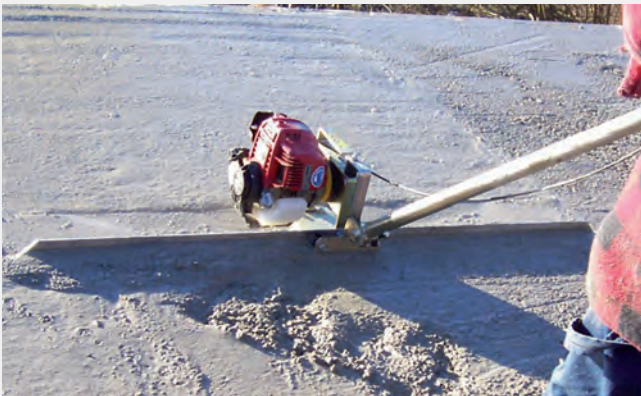
Scraping and compacting with scraper bars
