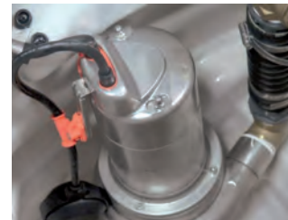
Pump with float switch
