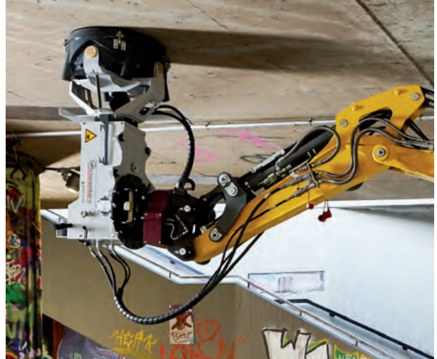
Working height depends on the length of the excavator arm
