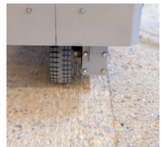
Milling of concrete and screed
