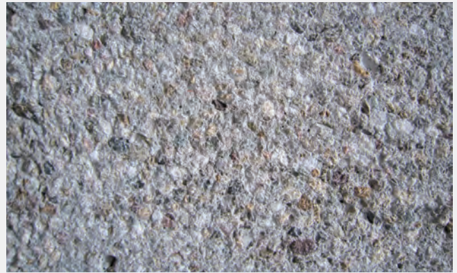
Scarifying results achieved during subsurface preparation
