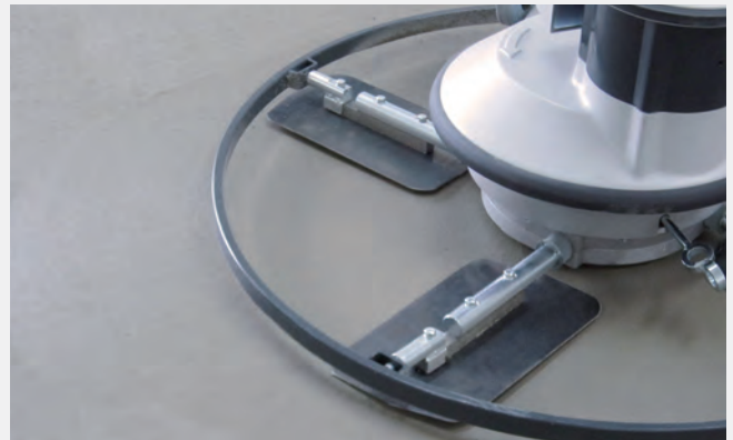
Smoothing with trowels
